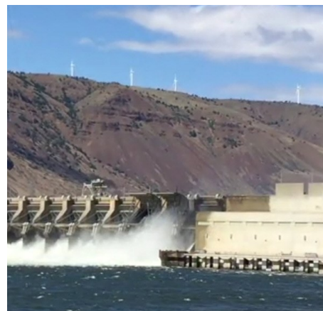
The John Day Dam and its substations comprise a primary pricing point for bilateral transactions involving output from hydroelectric and wind resources in central and eastern Oregon and Washington — often intended for delivery into California. | Oregon Department of Energy
